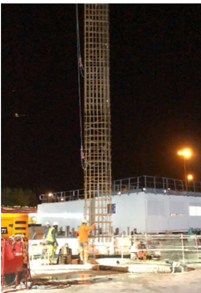
OA13 (line 15 of the Grand Paris Express) – installation of fibre optic cables in the reinforcement cage of a diaphragm wall
