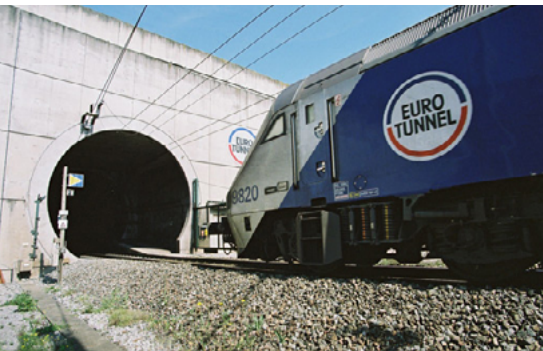
The entrance to the Channel Tunnel © Eurotunnel
